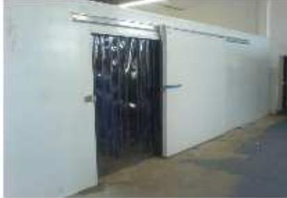
On bigger warehouse type cold freezer rooms the height of the cold freezer room is generally very high. It would be vital to select a thicker insulated panel for more structural strength. The corrugated type of insulated panels that we manufacture is becoming very popular in factories.
